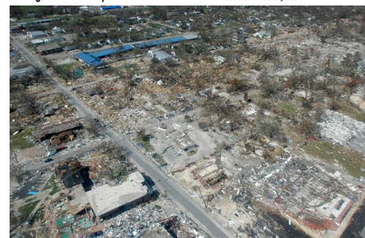
Wind and Storm Surge Damage in Gulfport, Mississippi
